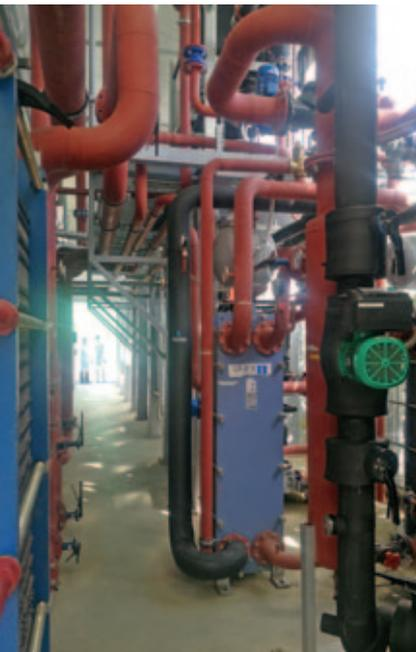
Originally the company used to utilize geothermal energy (installed capacity of 2,7 MW) for heating green houses with heat exchangers in addition to gas furnace installed capacity of 6 MW.
